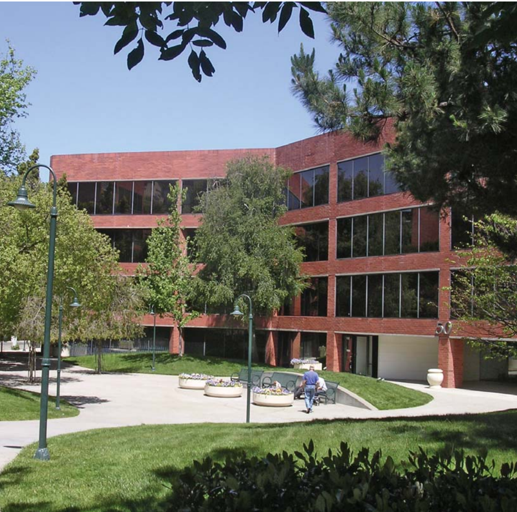
TEAMWRKX helps magazine magnate expand its West Coast office suite at 50 Francisco Street, Port of San Francisco
